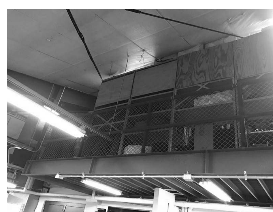
EXTG HEADHOUSE MEZZANINE: NEW FP EXPOSED.
