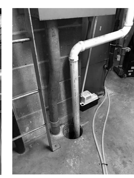
EXTG 1970s BDG L-2 CLOSET CORE DRILL FOR FP ROUTING.
