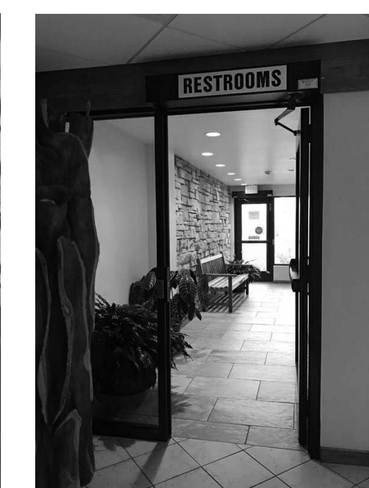
EXTG 1990s RESTROOM BLOCK HALLWAY: CEILING TO REMAIN AS IS.
