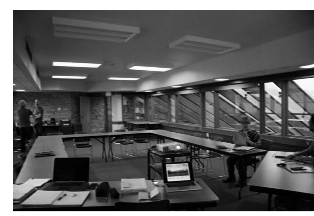
EXTG 1970s BDG L-2 CONF. ROOM: NEW FP IN EXTG CEILING.
