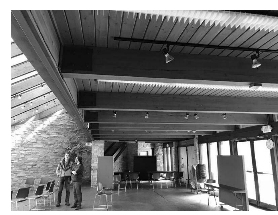
EXTG 1970s BDG L-2 HALLWAY: NEW FP IN EXTG CEILING.
