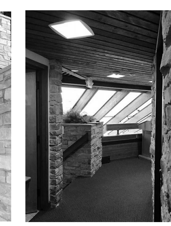
EXTG 1970s BDG L-2 HALLWAY: NEW FP IN EXTG CEILING.
