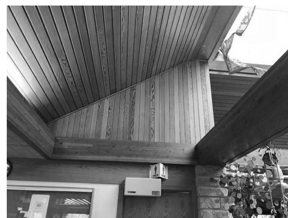
EXTG LOBBY RAKING WOOD CEILING TO REMAIN.
